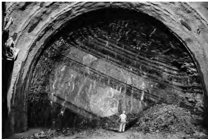
Figure 8. THE FACE OF THE VAGLIA TUNNEL IN THE MONTE MORELLO FORMATION (limestones, marls and sandstones).
