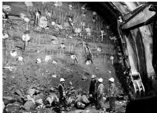
Figure 7. FIRENZUOLA TUNNEL: THE FACE REINFORCED WITH FIBRE GLASS STRUCTURAL ELEMENTS INSERTED INTO MICRO JET-GROUNDED COLUMNS.
