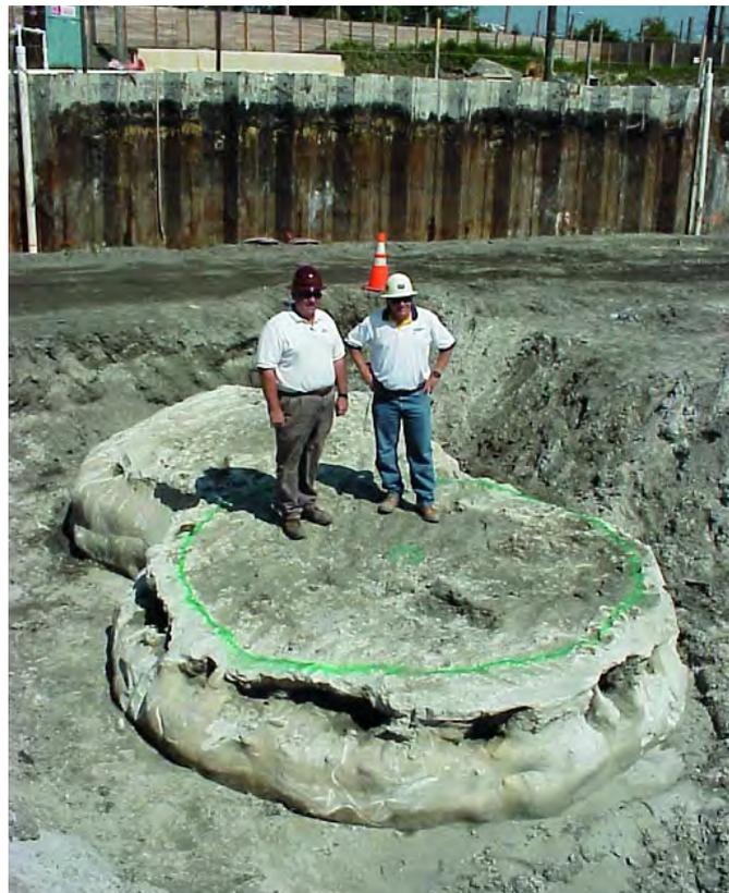
Foto No. 1. SUPERJET-GROUTING, COLUMNAS DE GRAN DIÁMETRO.
