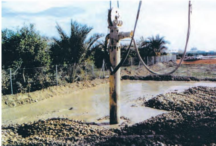
Figura 4. COLUMNAS DE GRAVA EN VÍA HÚMEDA (Keller Group, 2000).
