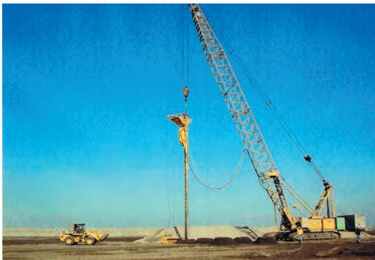
Figura 11. COLUMNAS DE GRAVA HASTA 37 m POR EL SISTEMA S-ALPHA DE KELLER (Keller Group, 2005).
