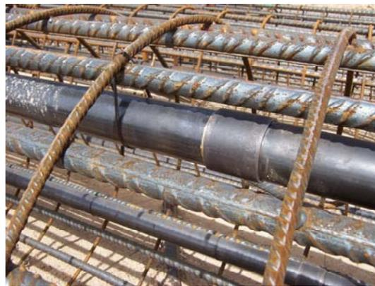
FIG. 2.14 TUBOS METALICOS INSTALADOS EN LAS ARMADURAS
