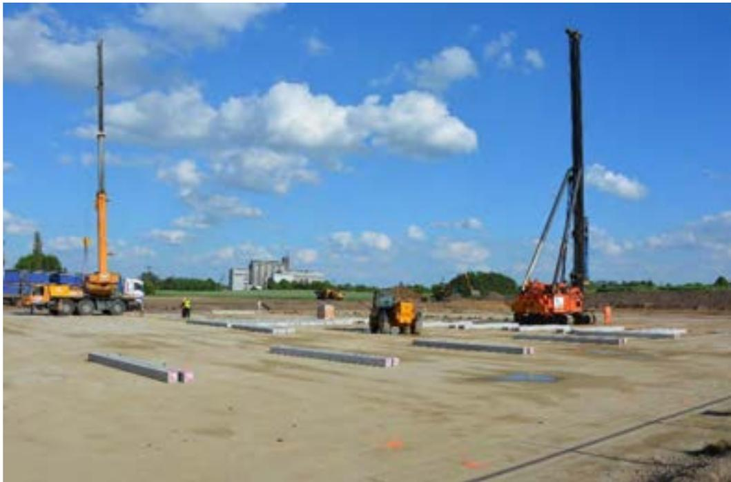
Fig A6. Example of a cement bound platform
