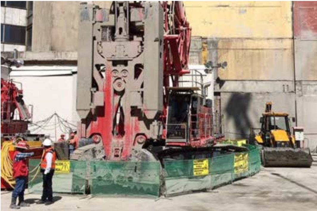
Fig A3. Example of a concreted platform
