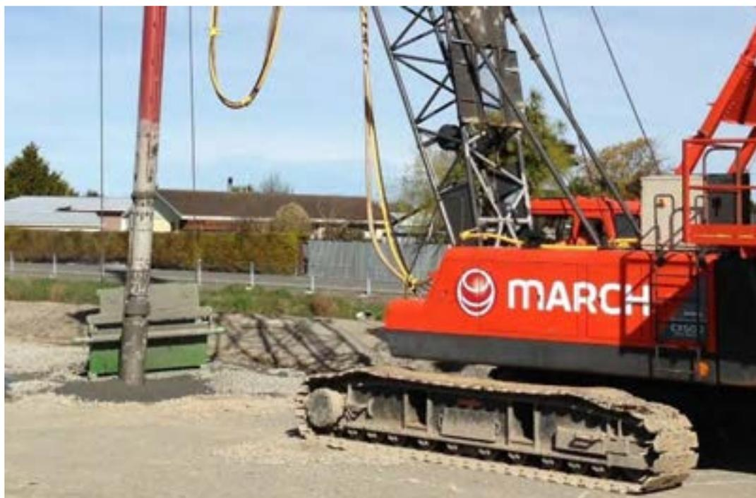
Fig A2. Well compacted granular platform
