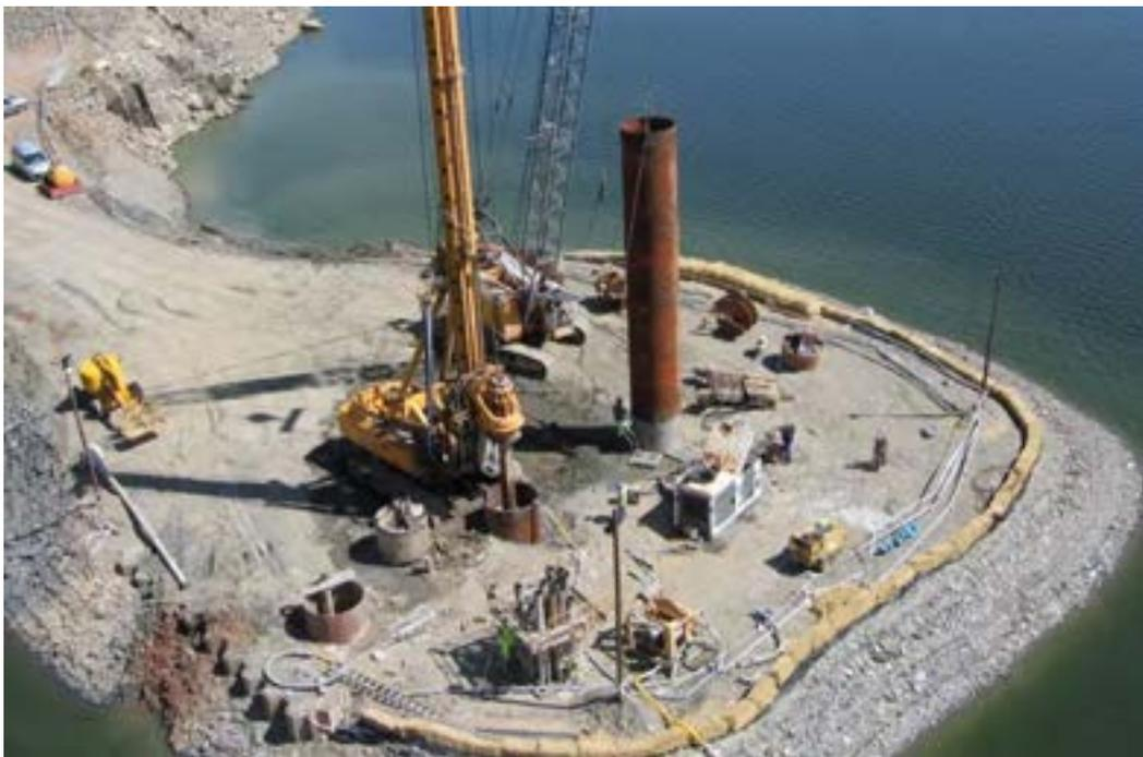
Fig A8. Example of edge protection around the platform
